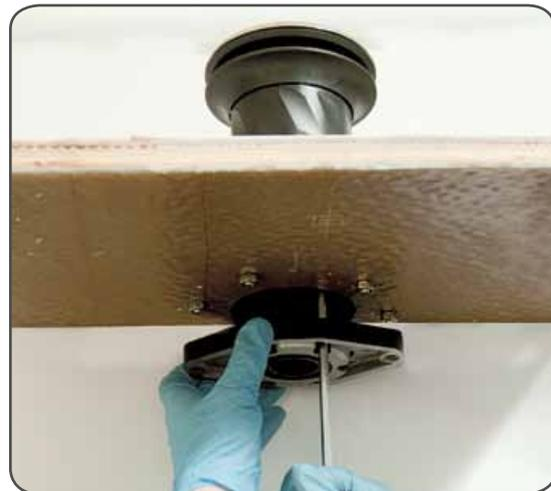
2. Tighten the six screws (8 Nm/ 71 in-lb)
